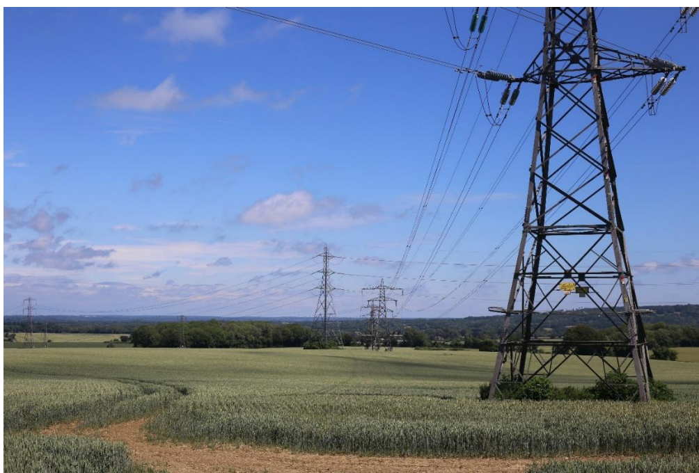
Plate 4: View of overhead lines and pylons across arable fields with distant views across the rolling landscape
