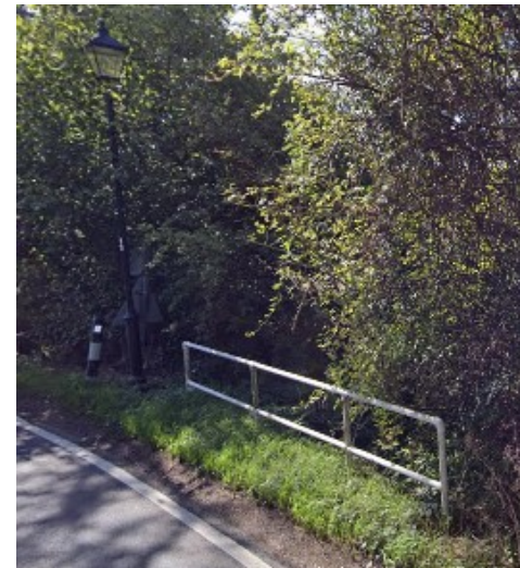
The utilitarian balustrade to the River Hart on Crondall Road with an adjacent “Windsor” style heritage lamp
