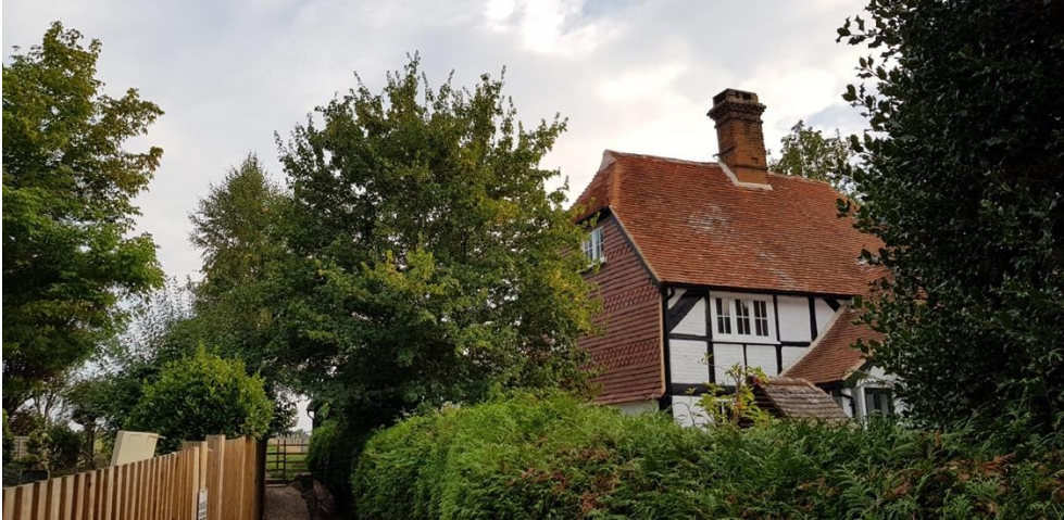
Figure 45 - Footpath 1 alongside Forge Cottage
