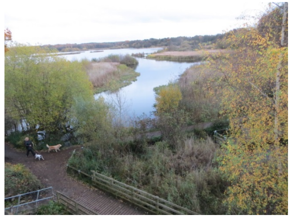
Fleet Pond – A natural reservoir where sensitive management of surrounding land is required.
