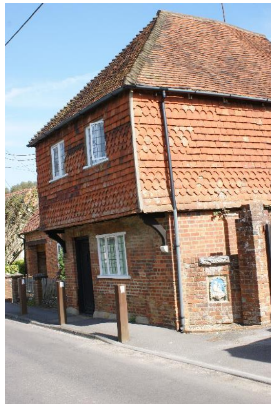
Figure 5 Manor House, Dippenhall Street
