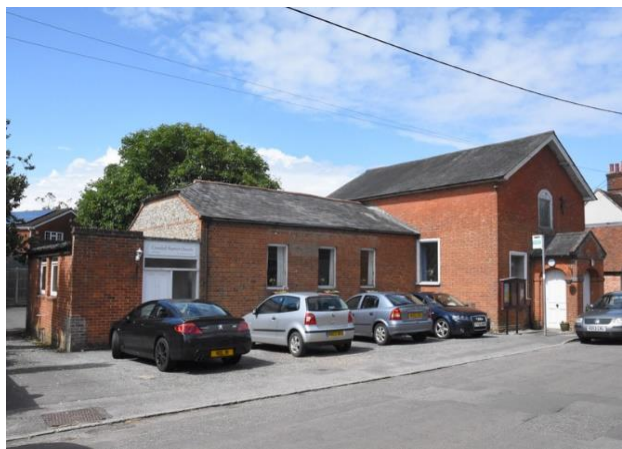
Figure 34 New Life Church and Car park
