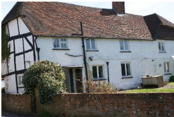
Figure 24 The Brambles, Timber Framed
