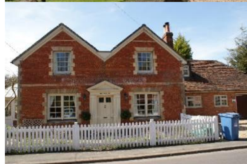
Figure 28 Chilloway Cottage and The Old Inn have both recently (2015-16) had side extensions
