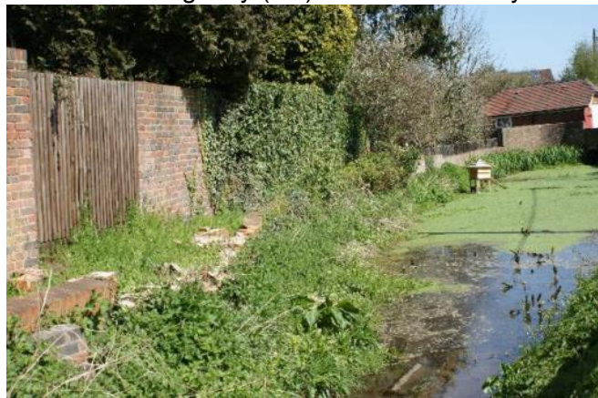
Figure 35 The Pond. Note damage to rear retaining wall
