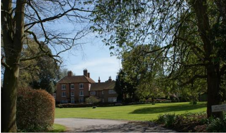
Figure 26 The Court, now divided into apartments
