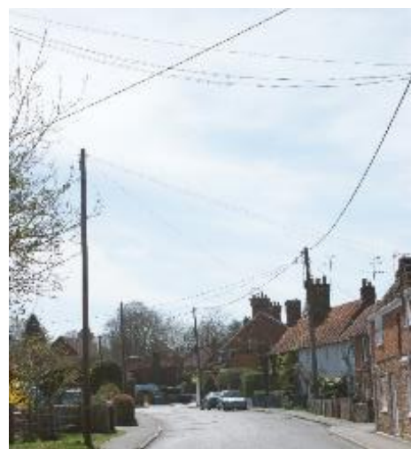
Figure 31 Overhead cables blighting the street scene
