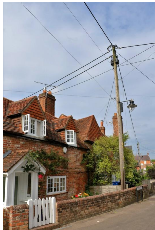
Figure 15 Heritage Lamp on telegraph pole. Note unsightly wires
