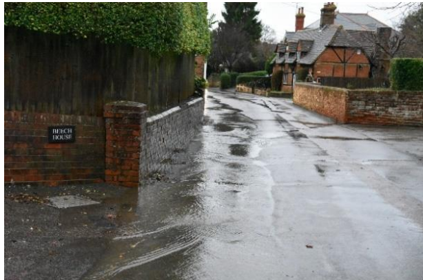
Figure 44 Surface water flooding in Dippenhall Street
