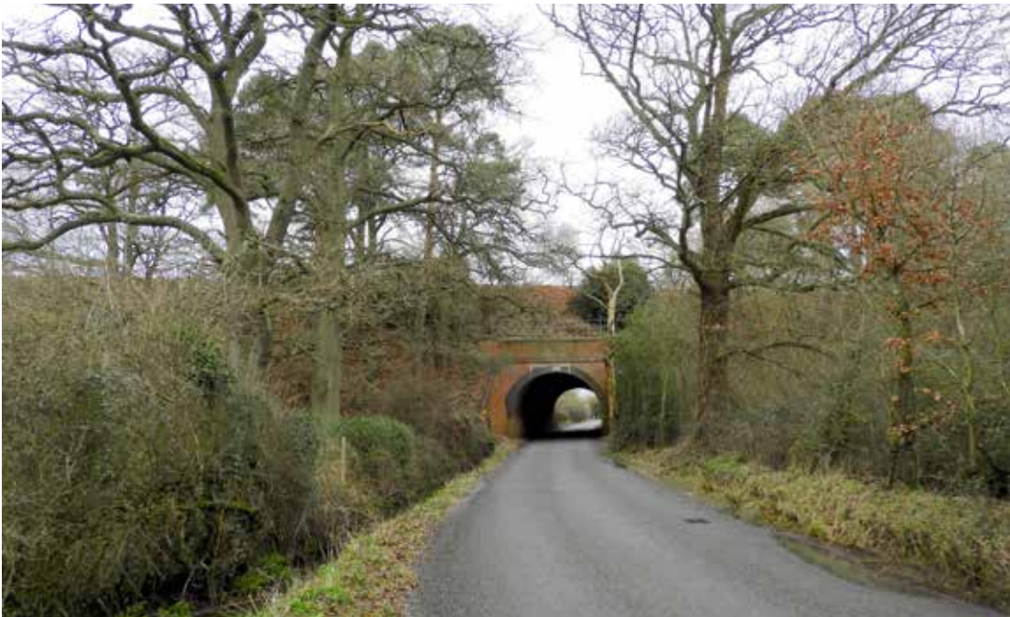
Railway bridge on Taplin's Farm Lane
