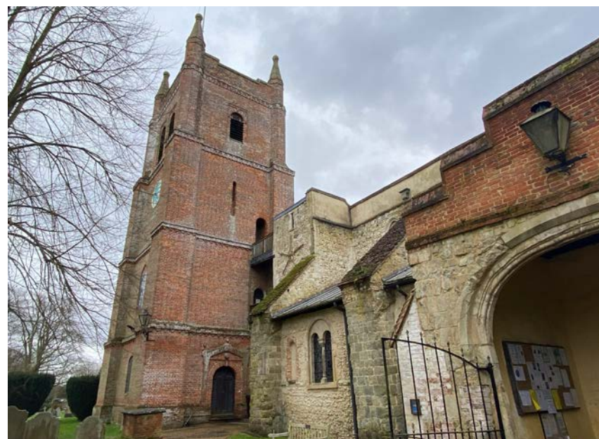
North elevation of All Saints' Church
