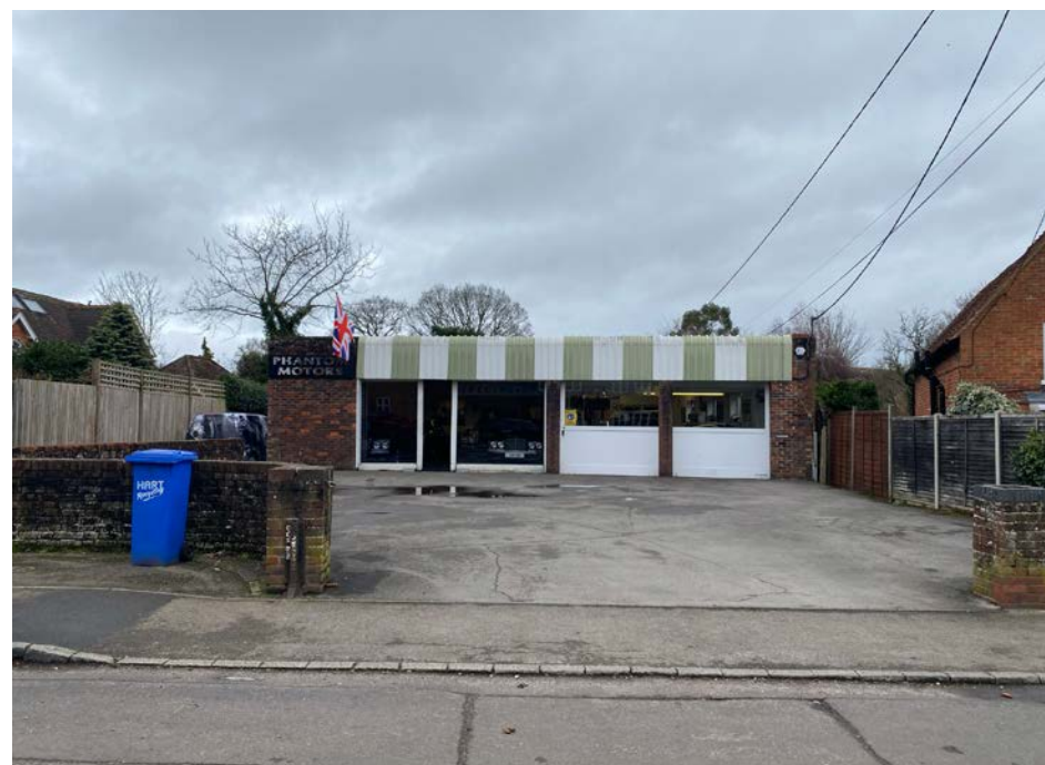
Phantom Motor Cars garage, Pankridge Street
