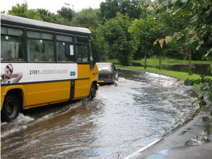
Figure 17 - Brandon Road balancing pond overflowed from a point close to its northeastern corner (July 2007).
