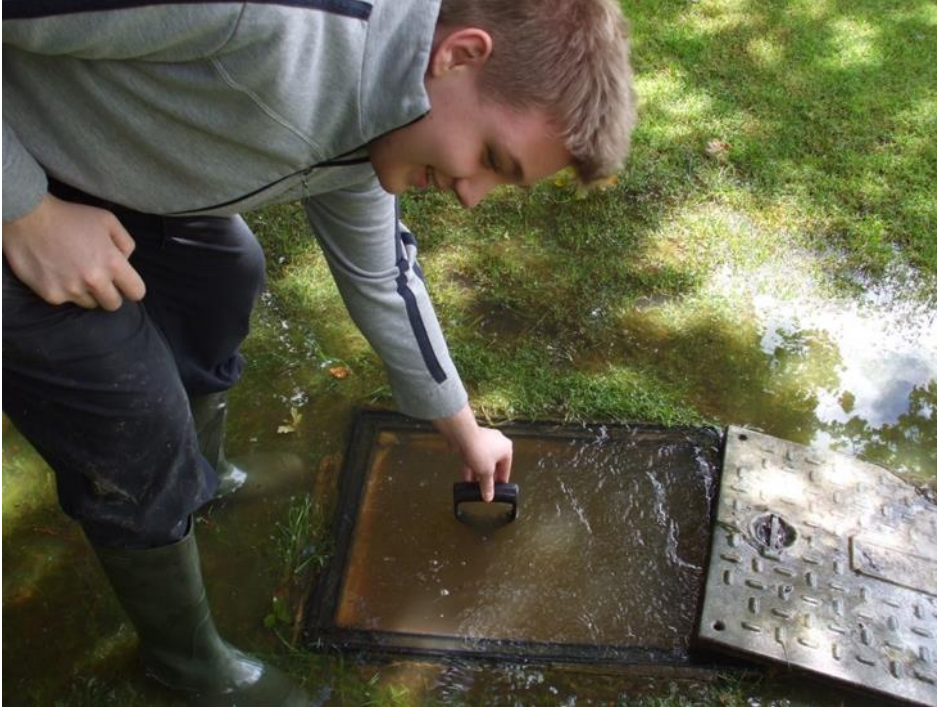
Figure 41 - Brooks Meadow - Adam inspecting flood water at drain cover
