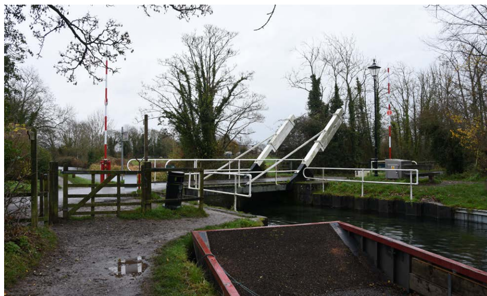
Swing Bridge over the canal
