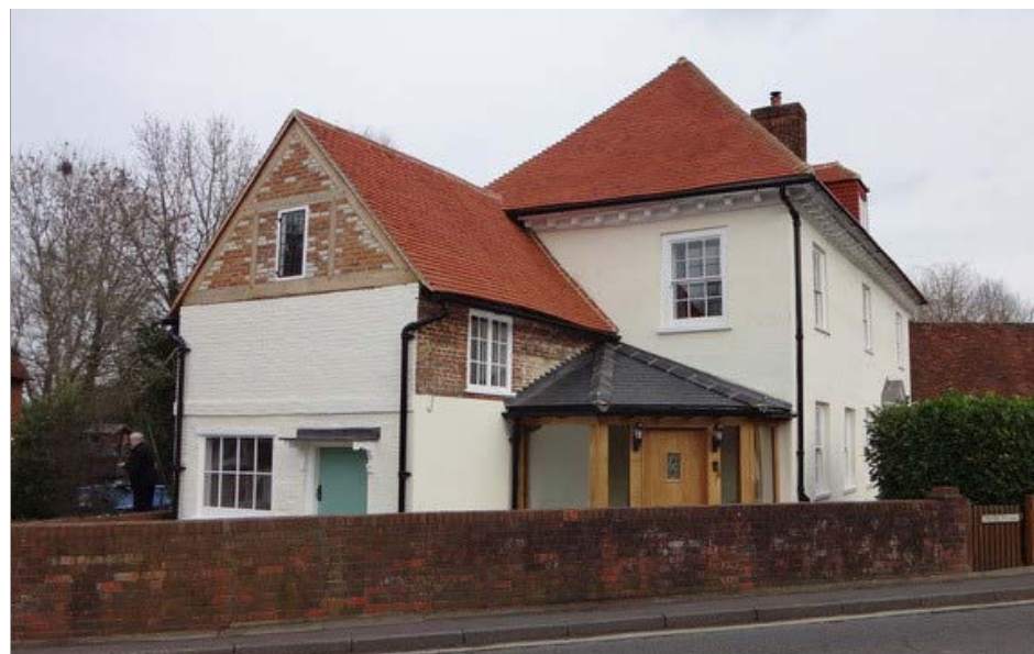
Timber framing on the side elevation and stucco on the front elevation of Nevills, Hook Road
