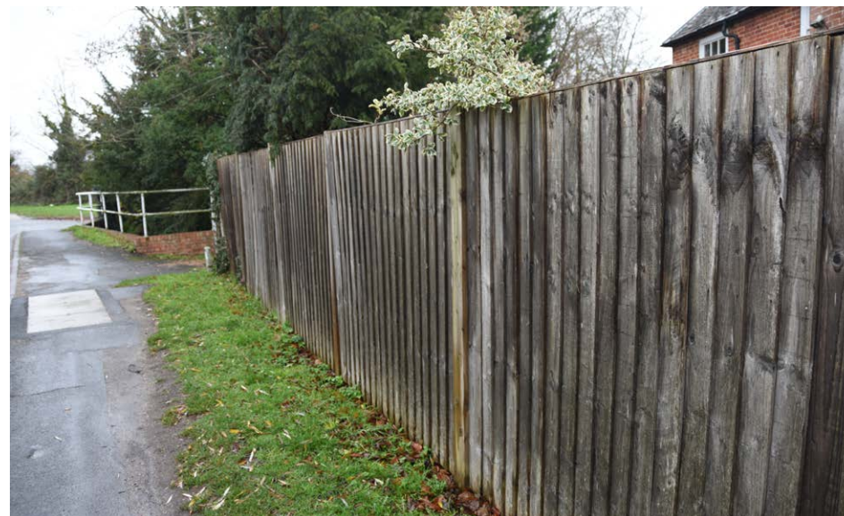
Tall close-boarded timber fencing on Hook Road and inappropriate modern metal railing on the bridge behind
