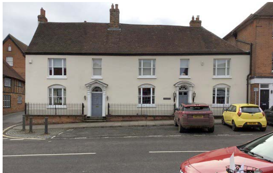
Nos. 67-69 High Street. The re-fronted north façade of a major 15th-century courtyard house
