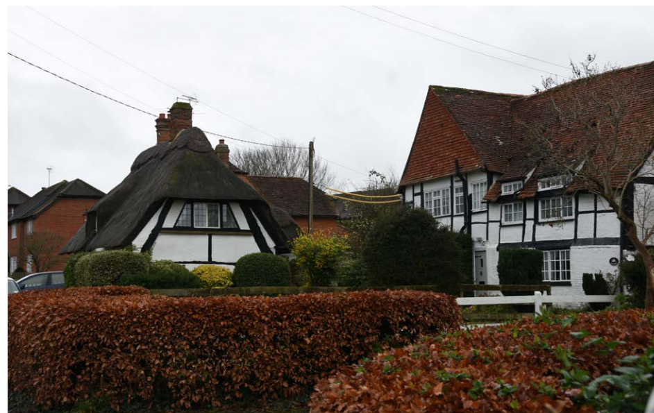
Cruck Cottage and Oakholme and Shepherd's Cottage, The Street
