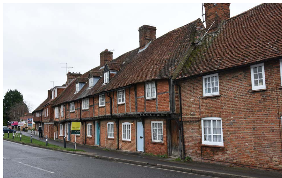
Castlebridge Cottages viewed from the south-west
