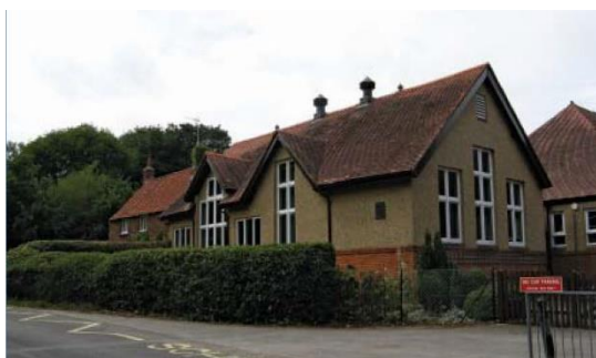
Rotherwick Primary School
